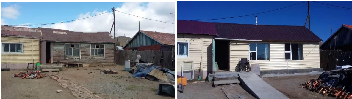
Complete renovation of a home
