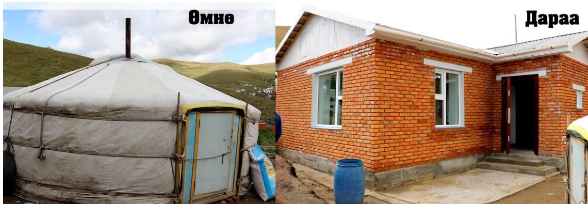
Construction of a pilot house for a family with a disabled child
