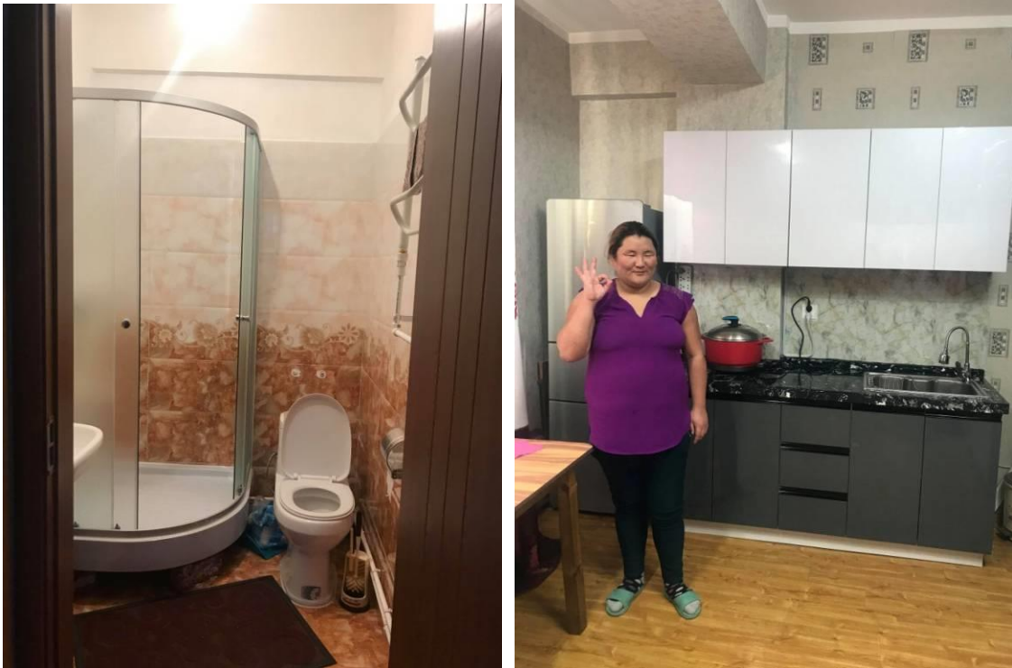
Illustration of the work carried out (new bathroom and fitted kitchen)
