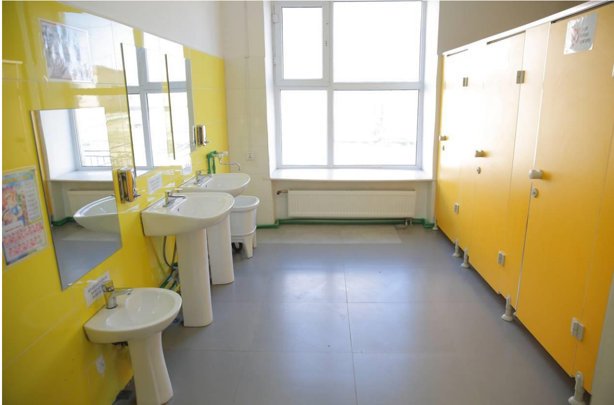
New boys' toilets at Bayankhangai school
